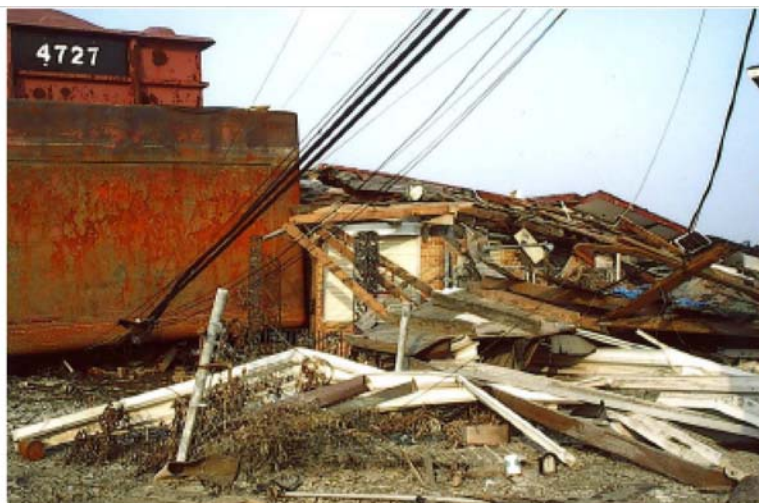
Figure 118: The barge adjacent to a semi-standing house (1739 Jourdan Ave.), which indicated the barge did not impact the house very hard.
