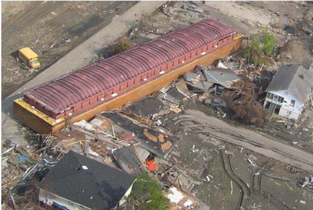
Figure 116: The barge in its post-Katrina resting place. The homes and trees would have prevented the barge from floating from the right side of this photo to its position on the left side of the photo, which is nearer to the canal.
