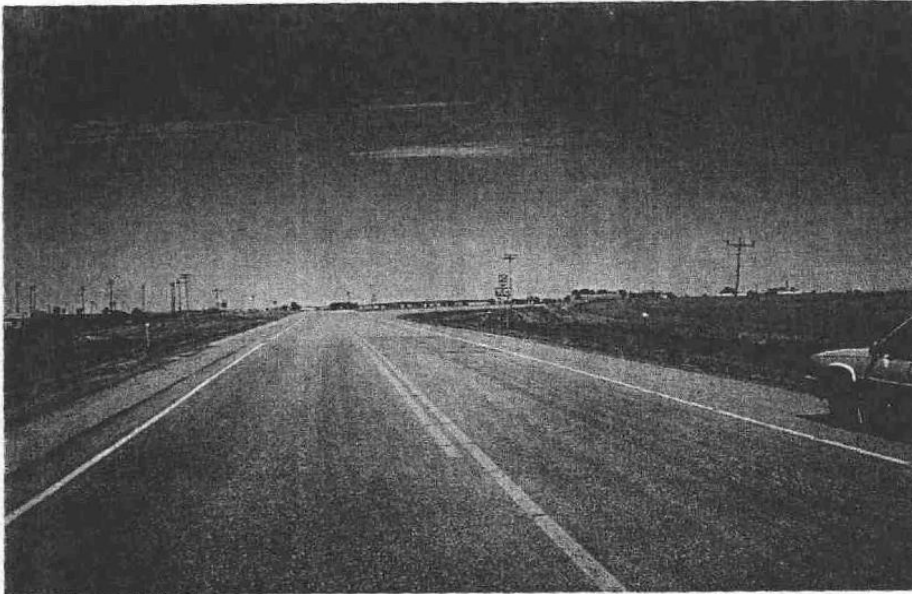
Photo No. 13 Date Taken: 8/30/04 Description: Approximately same view as #12 - Again shows double yellow & overall view of junction. Knoll on SE corner of junction in field partially hinders view of traffic from east.
