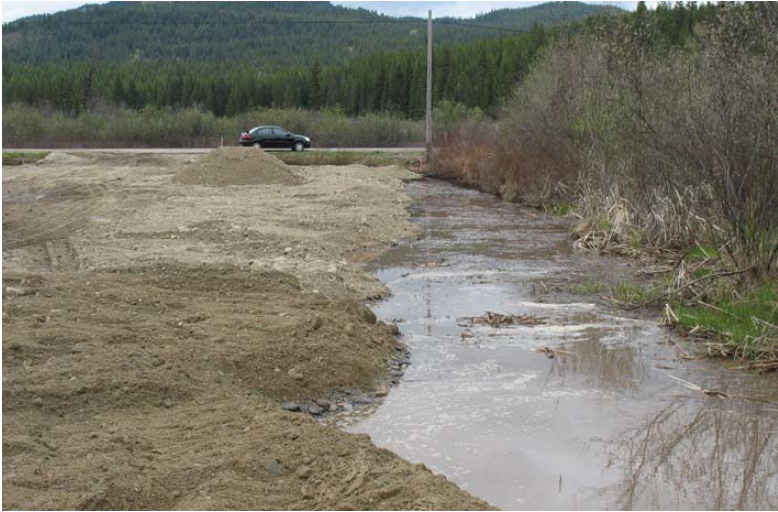
East side of the lot showing strip of excavated ground that was being filled when EPA officials arrived, taken during 2007 site visit.
