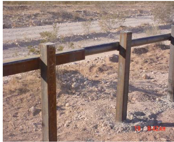
Photograph 2-1. Example of Post and Rail Vehicle Fence
