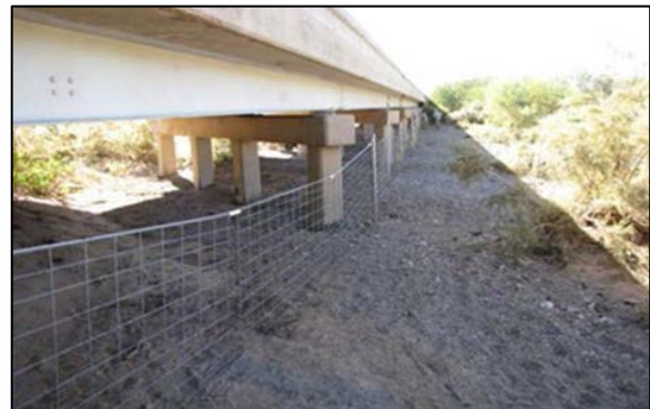
Figure 7.21: Example of strategic fencing being used at BMGR East to exclude trespass livestock.
