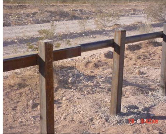
Photograph 2-1. Example of Post and Rail Vehicle Fence
