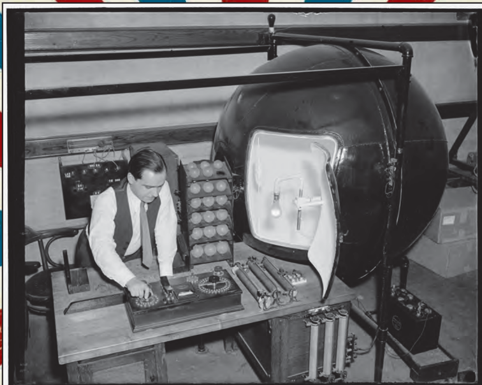
Test electric light bulbs for Uncle Sam. Purchasing on an average of 4,000,000 electric light bulbs annually, Uncle Sam is probably one of the largest users of light in the country. The National Bureau of Standards sees that the government gets value received in purchases by continually testing the incandescent lamps to determine their life and the amount of light they give. Using a special machine designed by the Bureau, Louis Barbrow is shown measuring the amount of light given by a lamp, 3/21/38, Courtesy Library of Congress, Photo by Harris & Ewing.
