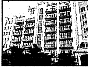
Project Front View
