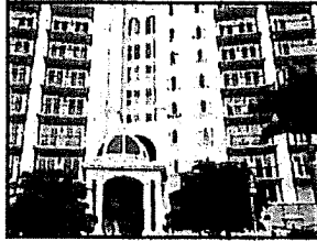
Project Front View
