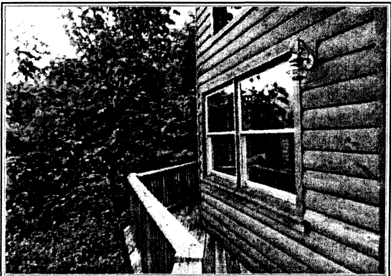
Addition Front View
