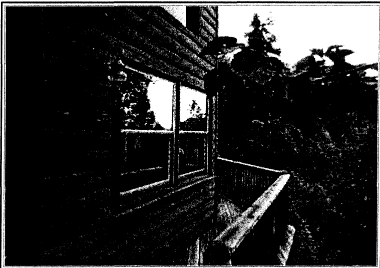
Addition Front View
