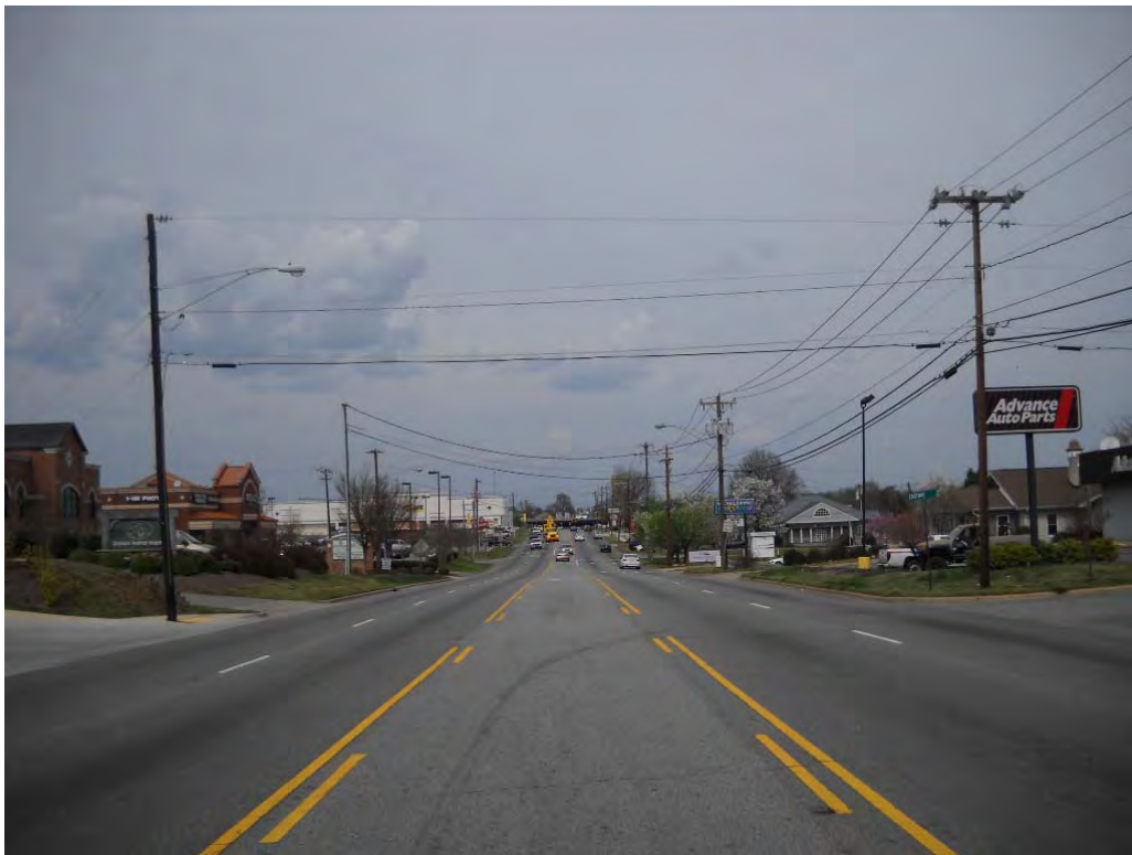
VIEW OF THE SOUTH MAIN STREET FRONTAGE
