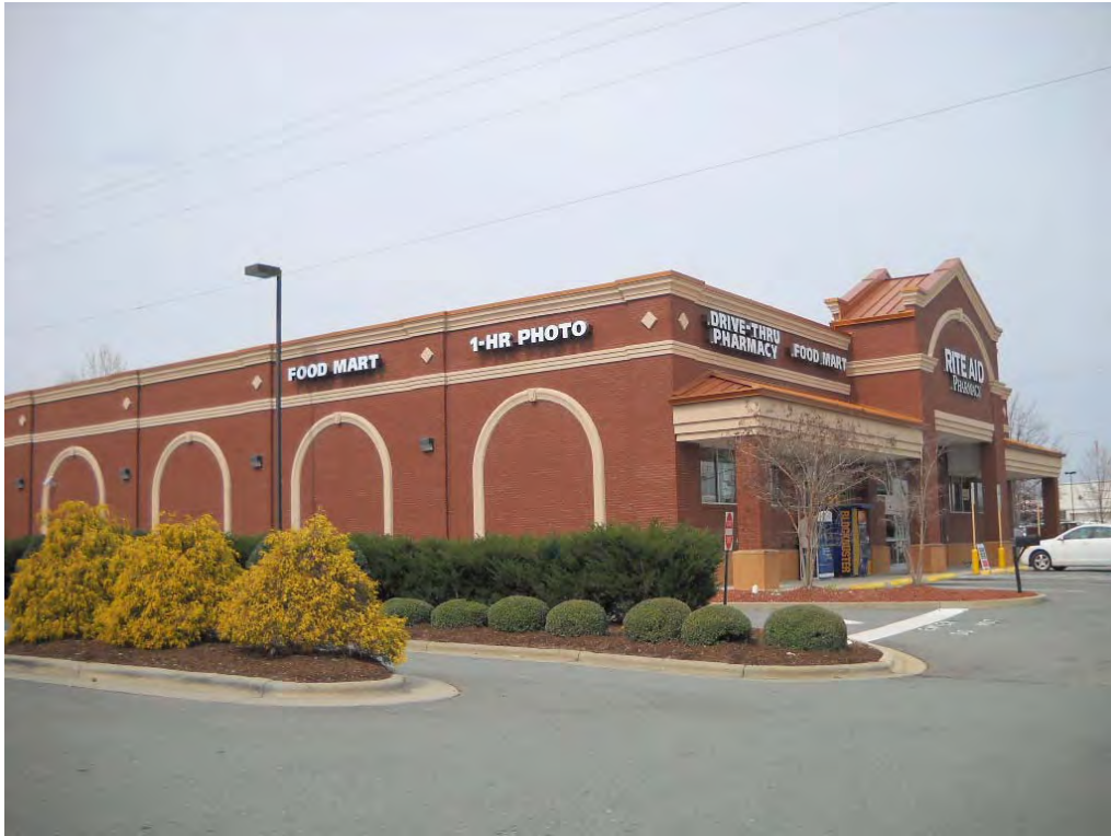
VIEW OF THE FRONT AND SIDE ELEVATIONS
