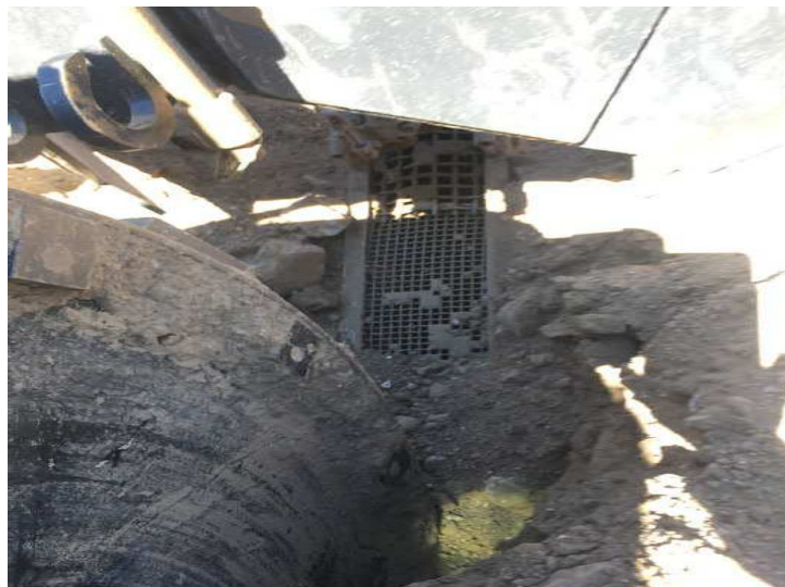
Photograph 8 – IMSG's Trenching System with Encasement Device
