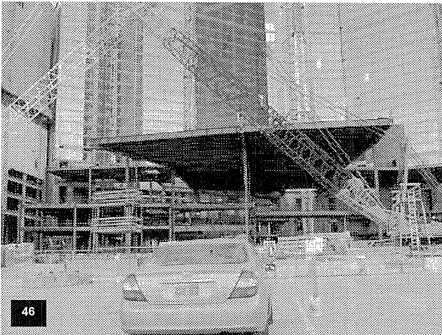
Podium – View of the structural steel framing of the Porte Cochere.
