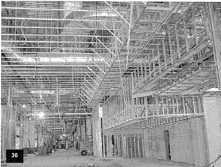
Garage/Convention Center – View of the service corridor for the meeting rooms.
