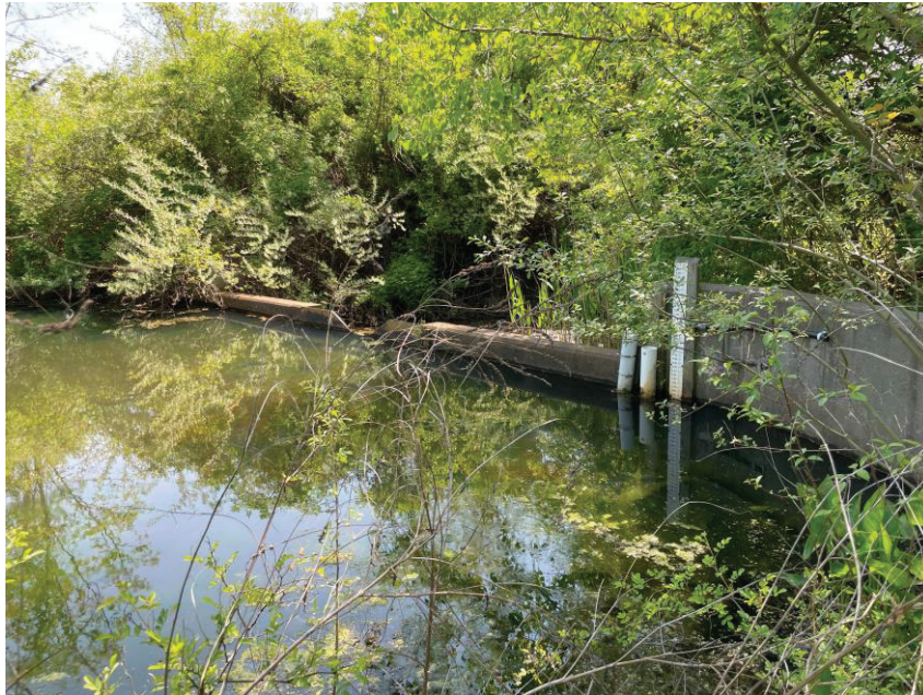
Figure 2: Existing Extended Detention Basin Outlet Weir
