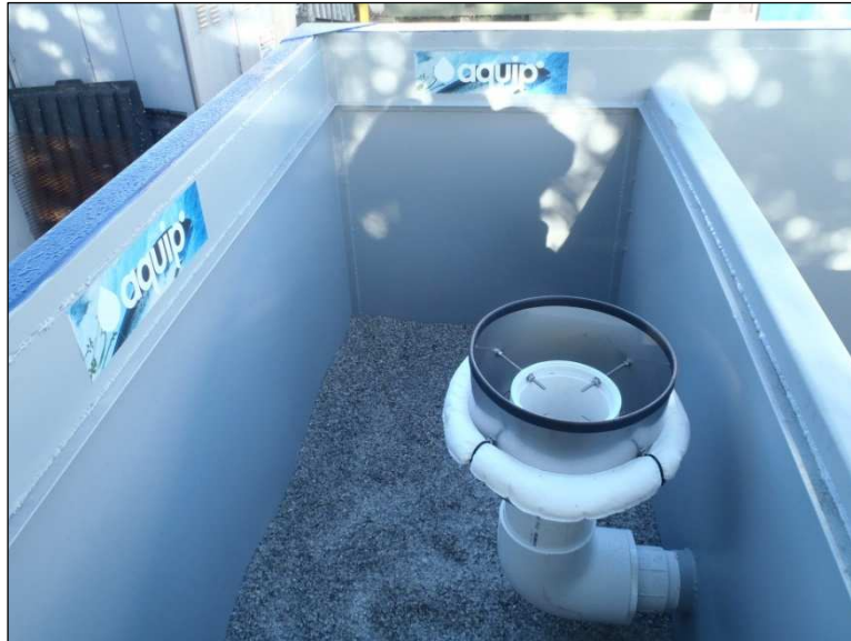
Figure 16. Pretreatment chamber oil skimmer sorbent pad.
