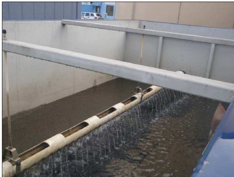
Figure 5. Best operating water level in filtration chamber for optimal pollutant removal conditions
