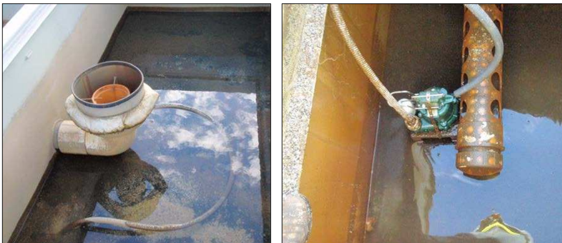
Figure 7. Aquip pretreatment chamber without pump (left) and with pretreatment pump (right).
