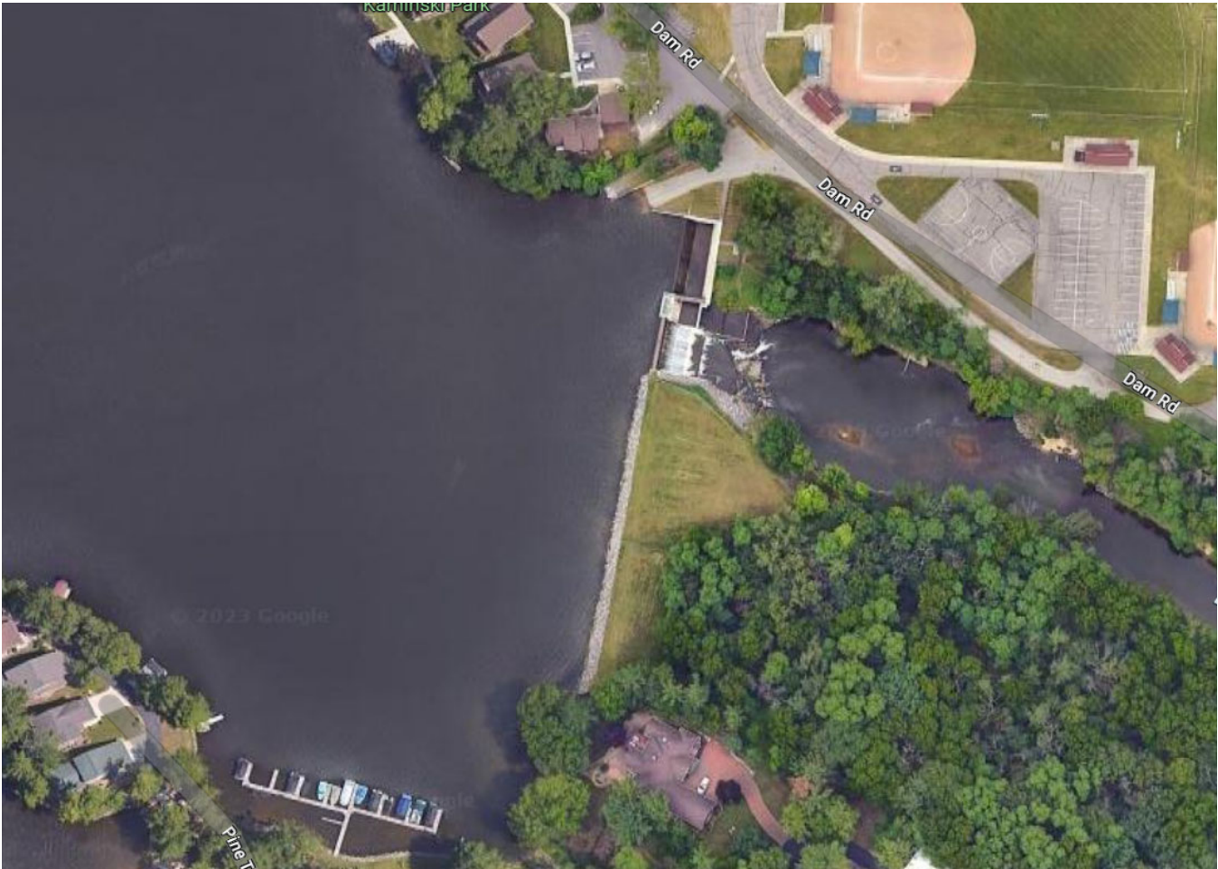
Google satellite view of the dam between Lake Delton and Dell Creek
