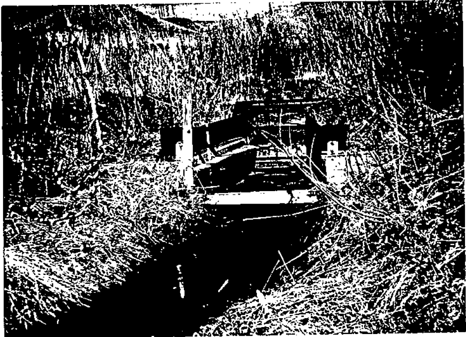
Photo No. 2. Photo Date: Early Spring 1990 Photo taken by Dan Voyich Subject: Parshall flume on Voyich Ditch.
