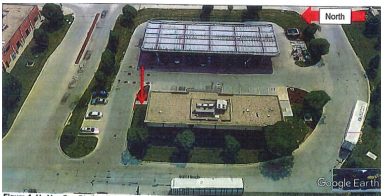
Figure 1. Hy-Vee Gas Station #10 looking east. Red arrow indicates location of air pump at time of incident. Via Google Earth.
