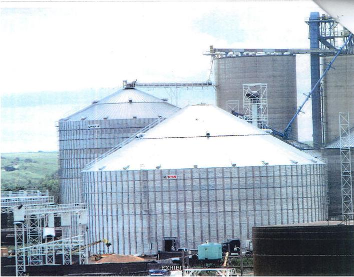
Construction on Ag Valley’s Edison facility was completed on November 1, 2007, and the Titan model CB50 was placed into service. Final payment on the construction project was made by Ag Valley to Heartland on November 30. The Titan model CB50 was full of grain when it collapsed without warning almost 10 years later, on August 6, 2017.
