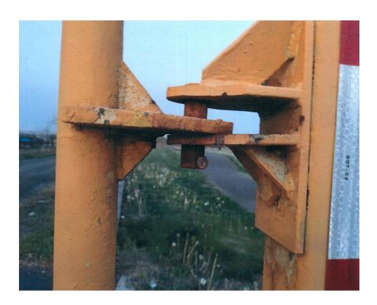
It is the parents' theory that the room on the pin for the gate to swing freely presents a hazard if children are playing on the gate. They contend that the weight of children climbing on the gate will cause the gate's connecting plate to move up, and when the children jump off the gate, the gate's connecting plate will drop back down, pinching any fingers that might be in the way. As their lawyer argued at the summary judgment hearing:
